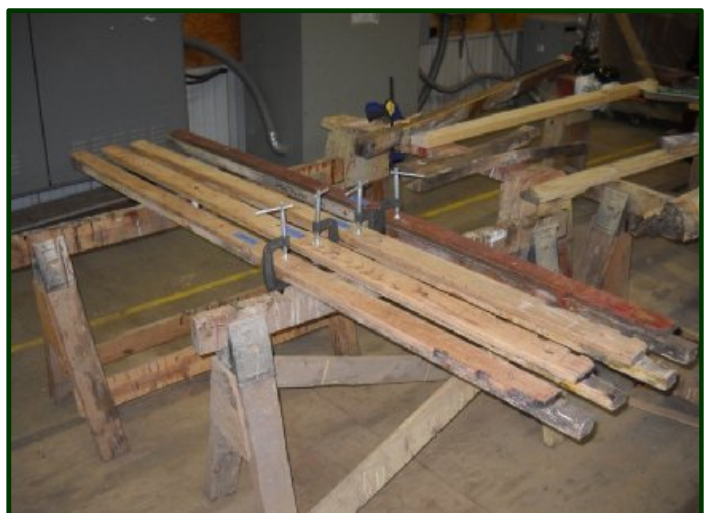
Repairs are being made to several of the platform end posts.
